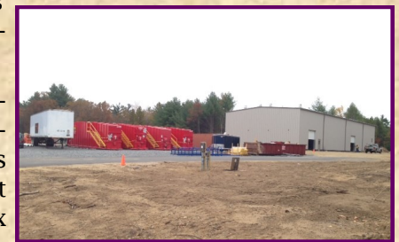
New treatment building
