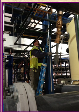
Tom Brosious works on level switches for the new concentration tank.
