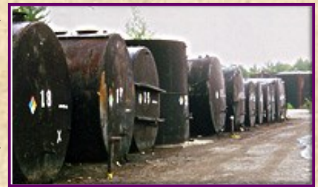
View of tanks on site prior to the EPA Removal Action
