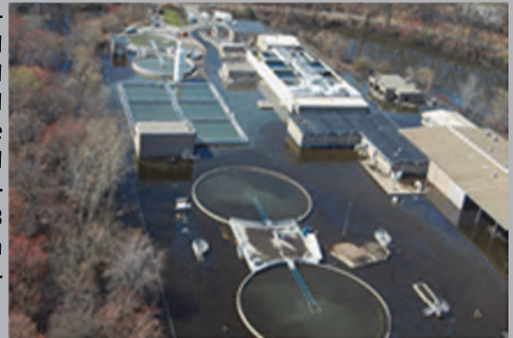
The West Warwick Wastewater Treatment Facility is submerged as a result of historic flooding.
