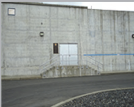
The flood high water line is marked with blue tape on the treatment plant exterior wall..
