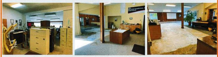
The final (and most disruptive) phase of our office renovation has now been completed. Over the course of several weeks, old carpeting was removed, concrete slab floors were leveled, and new carpet tiles were installed. The work was completed in stages as office furniture, computers, and other office equipment was temporarily relocated as the carpet installation progressed. We managed to remain fully operational despite not always knowing where our desk would be.
